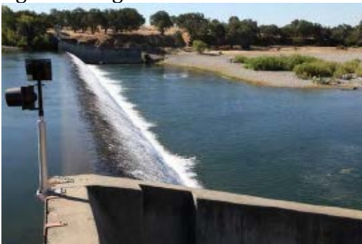
Figure 3. Daguerre Point Dam
